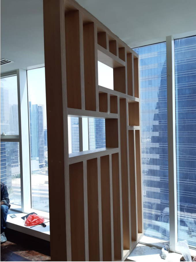
In-Progress Picture of Decorative wooden slat partition, Parquet flooring and Wall Cladding Works for Al Aber Contracting Chairman's Office in Business Bay, Dubai
