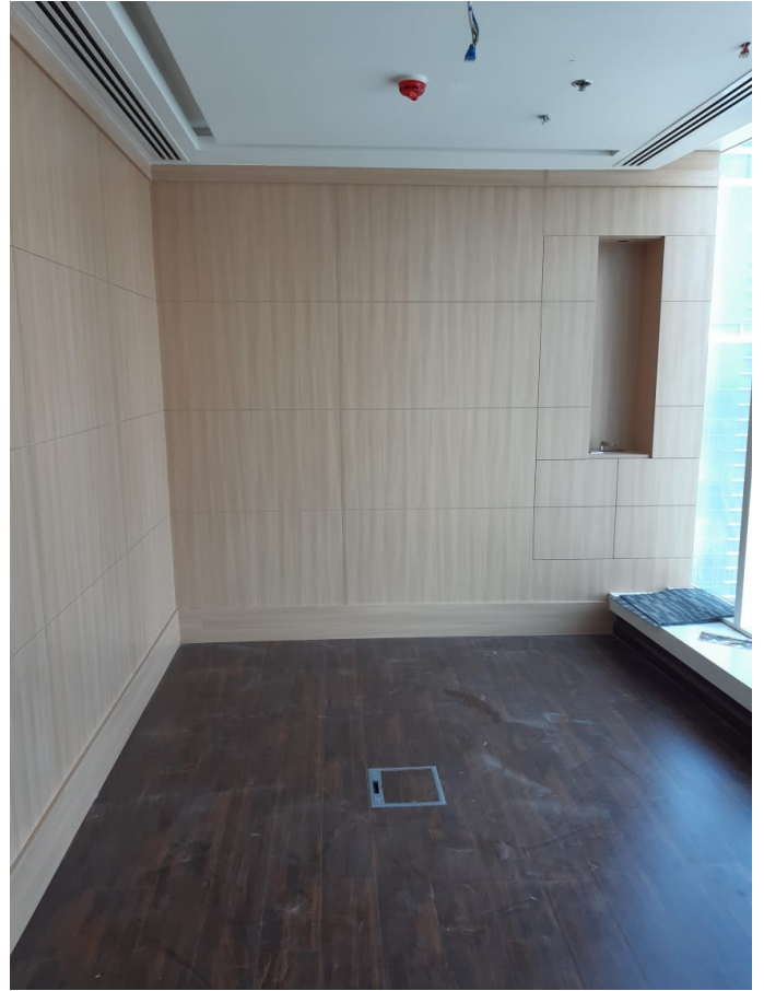
In-Progress Picture of Decorative wooden slat partition, Parquet flooring and Wall Cladding Works for Al Aber Contracting Chairman's Office in Business Bay, Dubai
